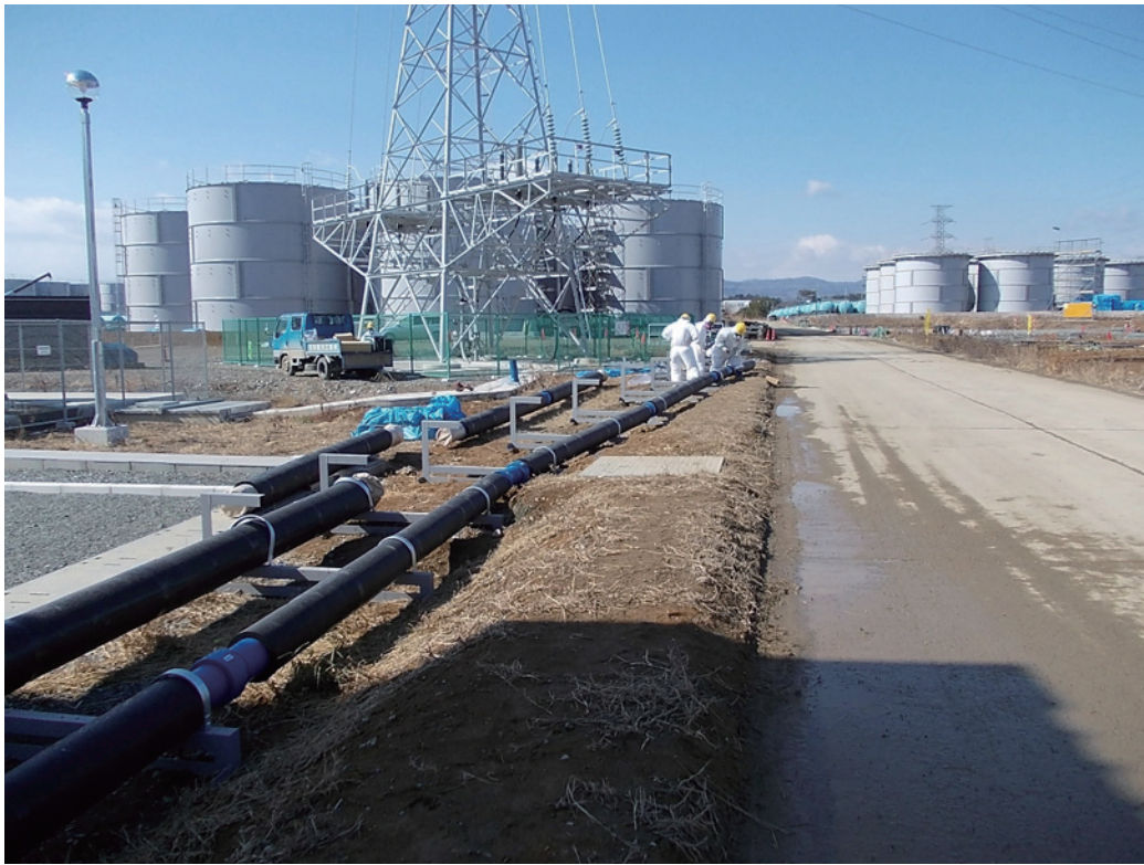
Figure 2. Some of the large number of storage tanks at Fukushima Daiichi Nuclear Power Plant (Photo by TEPCO)
